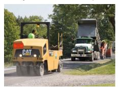
Chip Seal is a very cost effective means of Pavement Preservation. It typically costs one fourth to one fifth the cost of a conventional asphalt overlay. Chip Seals can extend the life of a roadway by 5-7 years as well as correct pavement conditions such as surface bleeding (where liquid asphalt leeches out of the pavement), variations to surface texture, raveling (disintegration of pavement due to loss of aggregate), cracks, decreased skid resistance, etc.
