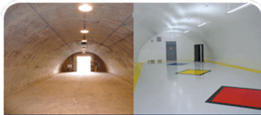
BUNKER INTERIOR - BEFORE AND AFTER
