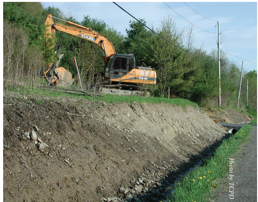
Ditch Grading in Tompkins County
