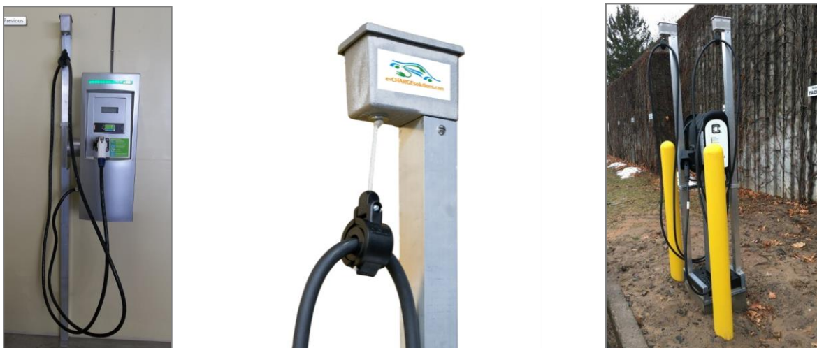
Figure 9: EV Charge Solutions EVSE Cable Management Examples 1
