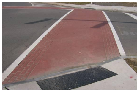
Example of a colored and textured crosswalk
