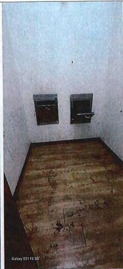
Figure 2b. Chute doors open. Trash room – 4 th floor.
