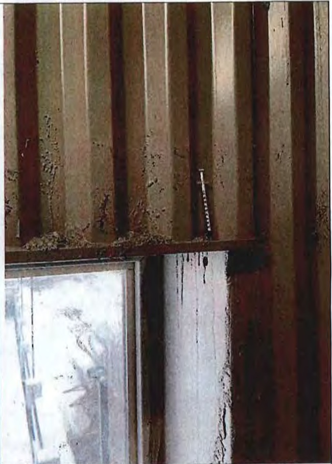
Figure 13b. Used hypodermic needle on landing between 9 th and 8 th floor. East stairwell.
