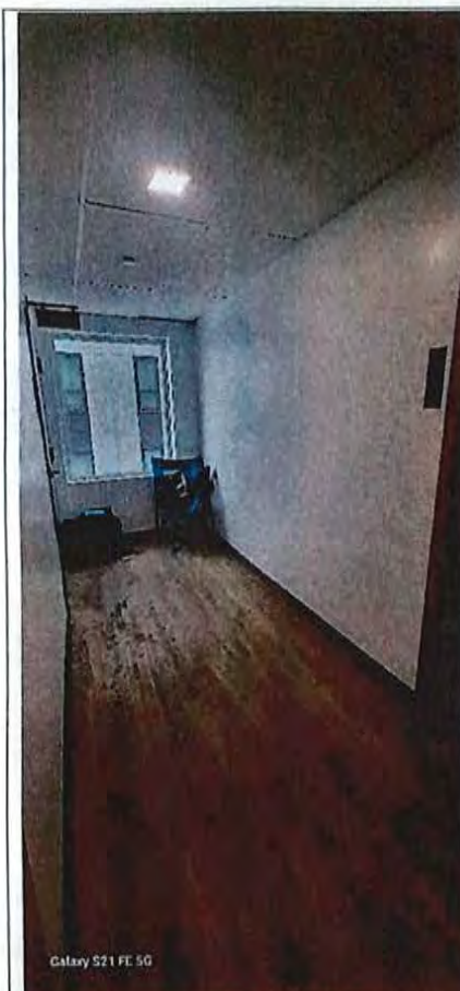
Figure 5a. Outside 7 th floor trash room (door locked).
