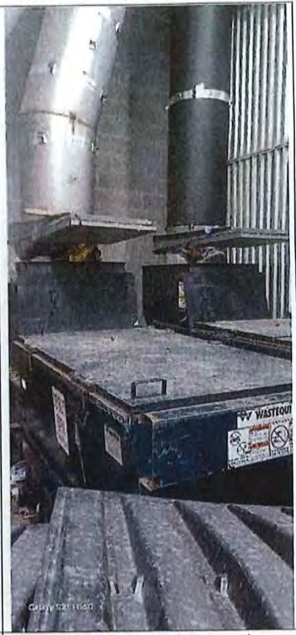
Figure 10c. Garbage chutes and trash compactors. Note: compactors filled to capacity and trash pick-up not scheduled until following morning.
