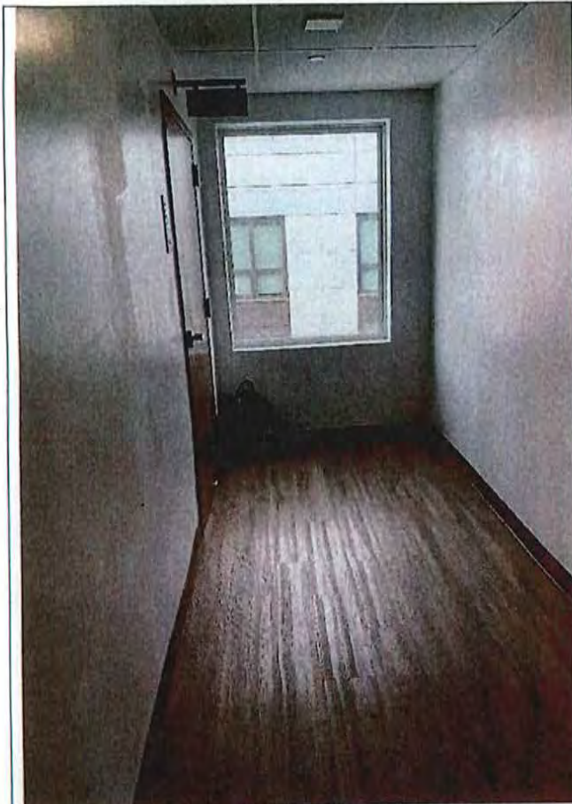
Figure 11a. Outside 12 th floor trash room.
