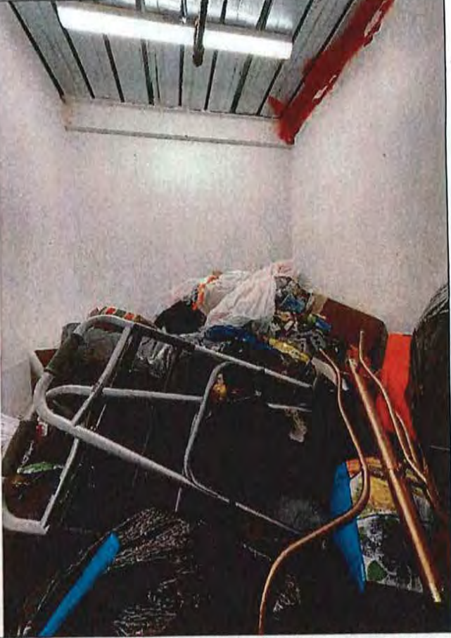
Figure 10b. 11 th floor trash room. Trash depth from floor approximately 5.5 feet.
