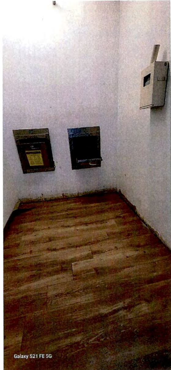
Chute doors open. 7 th floor trash room
