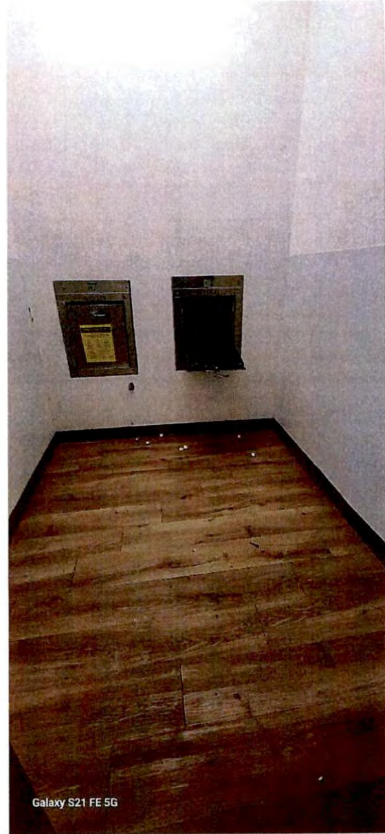
Chute doors open. 11 th floor trash room
