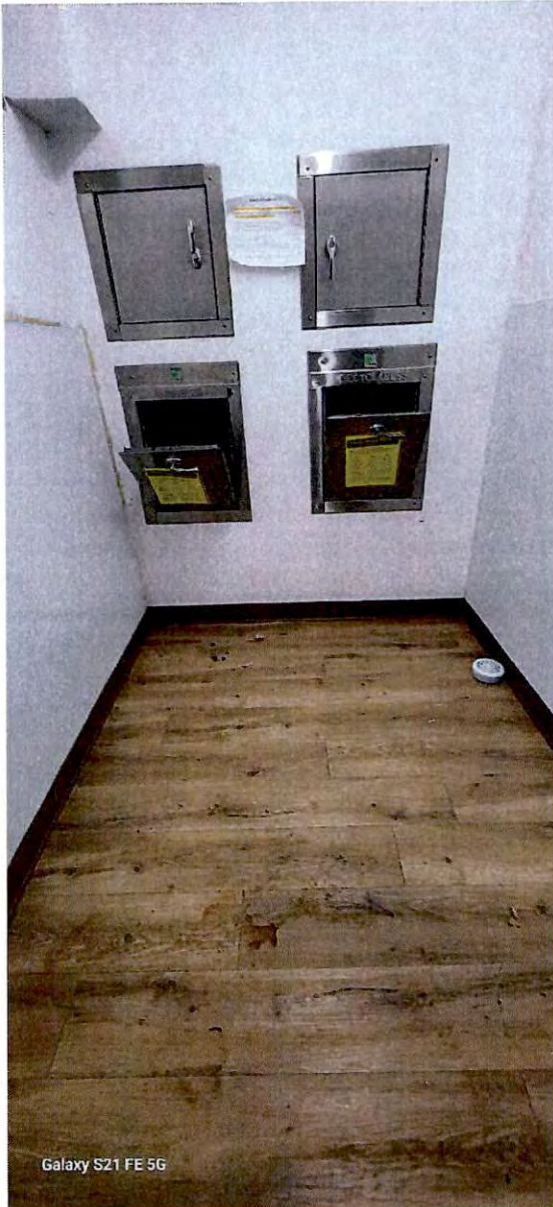
Chute doors open. 12 th floor trash room
