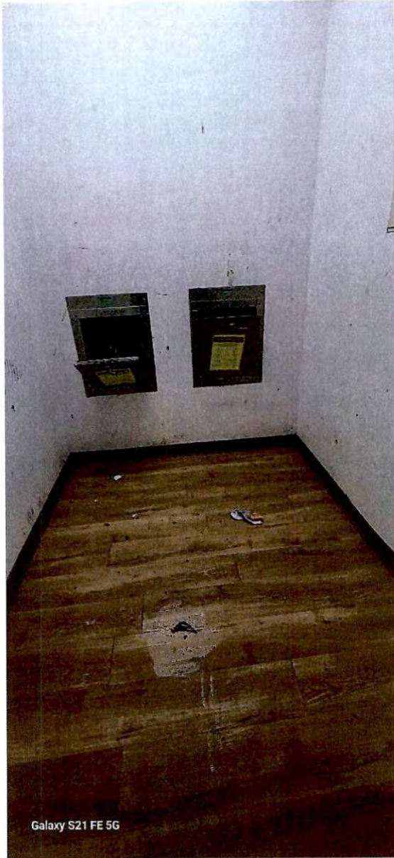
Chute doors open. 6 th floor trash room
