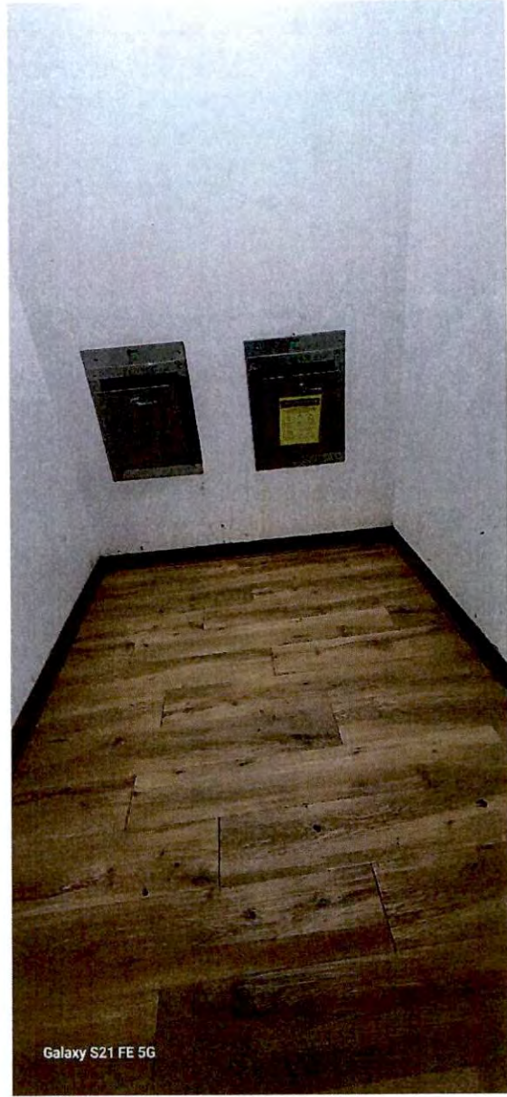
Chute doors open. 8 th floor trash room
