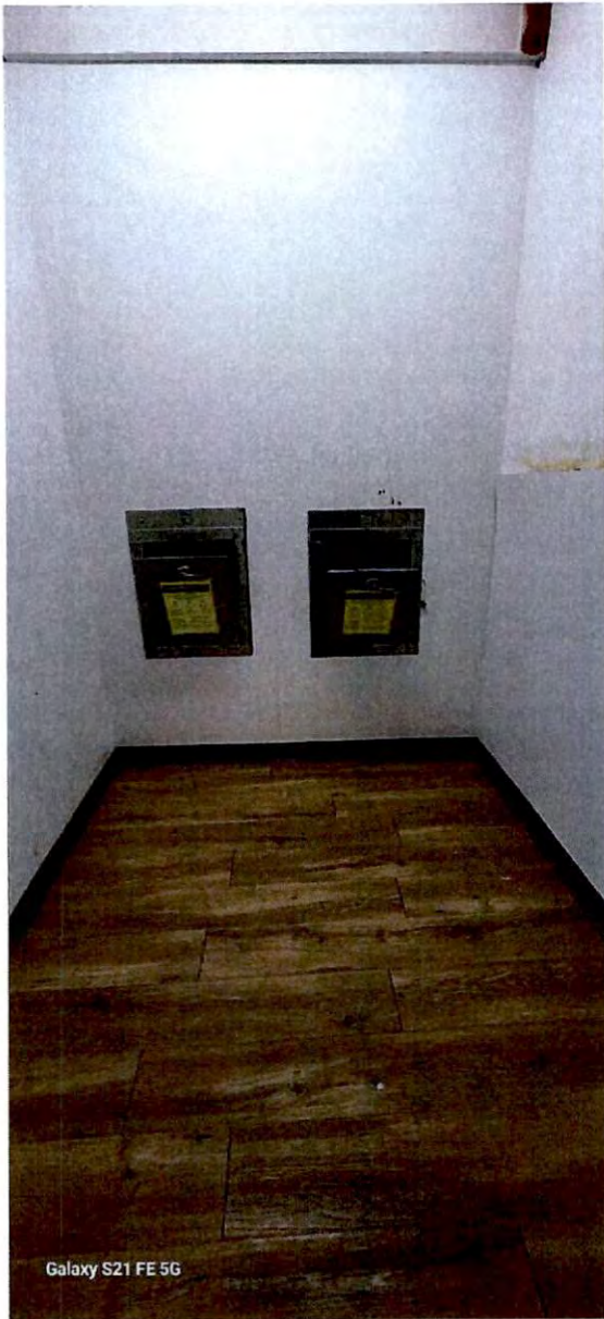
Chute doors open. 9 th floor trash room
