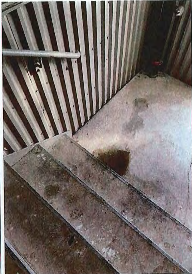
Figure 5a. Urine. Stairwell landing between floors 7 and 8.
