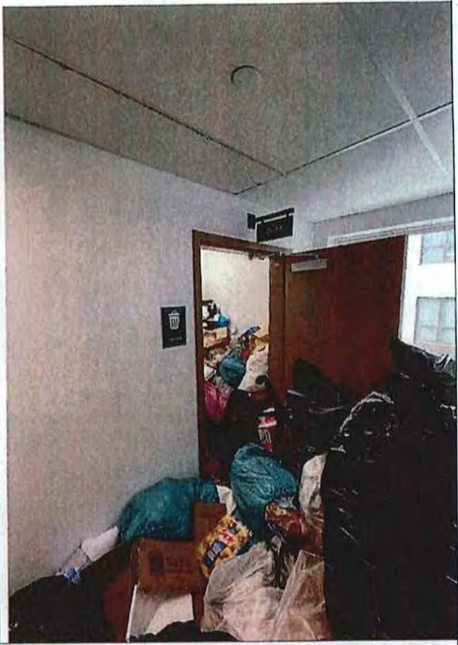
Figure 8b. 10 th floor trash room – refuse piled over 6 feet from floor.
