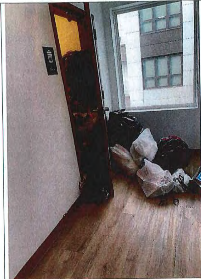
Figure 10a. Outside 11 th floor trash room.
