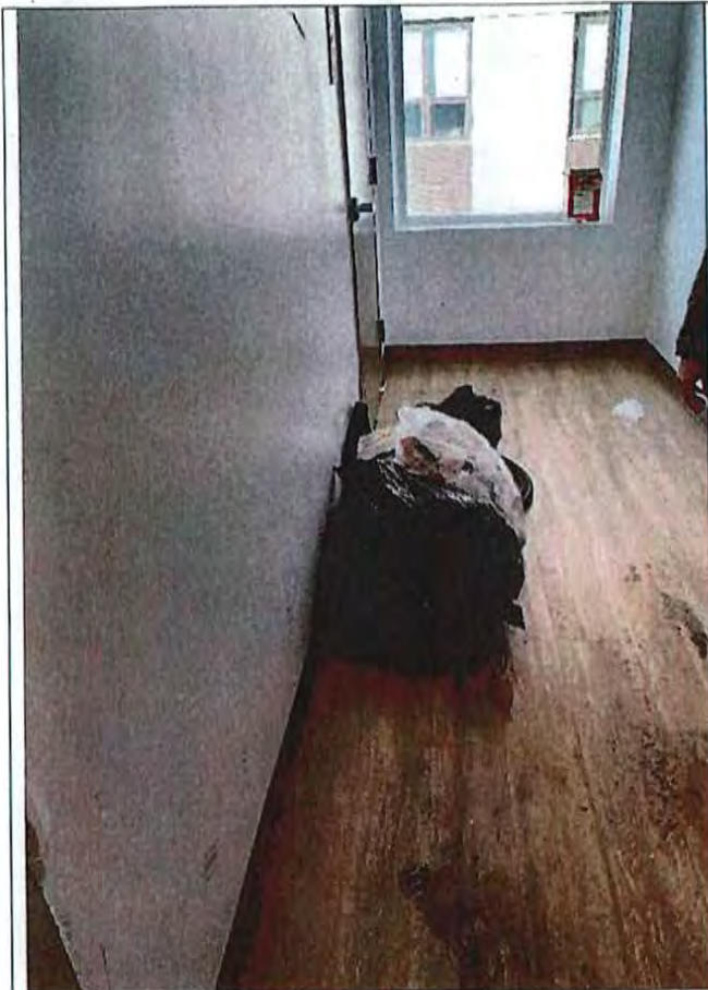
Figure 2a. outside 5 th floor trash room.
