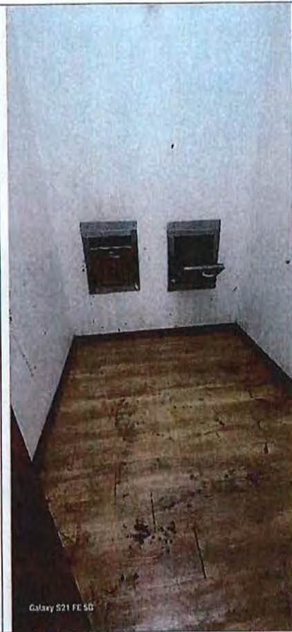
Figure 2b. Chute doors open. Trash room – 4 th floor.
