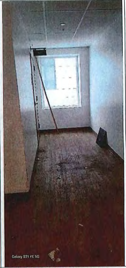
Figure 4c. Outside 6 th floor trash room (door locked).
