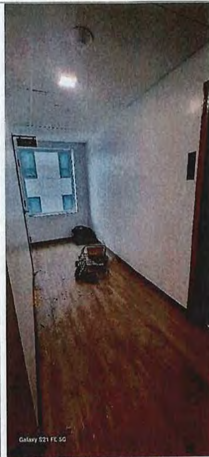
Figure 5c. Outside 8 th floor trash room (door locked).
