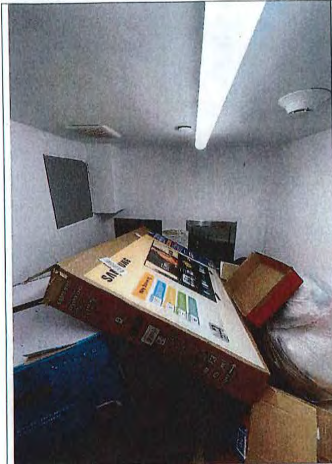
Figure 12a. 12 th floor trash room – chute doors closed.
