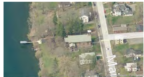
Aerial view of the Dublin Rd ROW
