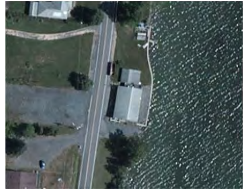
Aerial view of Wolff's Grill and Marina
