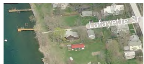
Aerial view of the Lafayette St ROW
