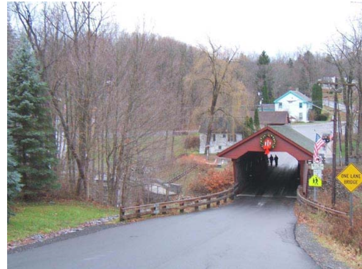
View D6 of the Newfield Covered Bridge is found on Bank Street near its intersection with Bridge Street in the hamlet of Newfield. The photograph is looking E and the view is approximately 45° wide.
