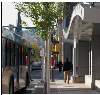
Highly utilized transit stops may include a building with amenities, such as restrooms and newsstands (far left). Smaller stops can be incorporated into the architecture of a building, and still offer shelter and relief from the elements (left).
