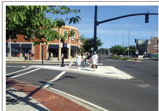
Figure 5. A pedestrian refuge at a channelized right turn to accommodate large vehicles. Source: Dan Burden, Walkable Communities, Inc.
