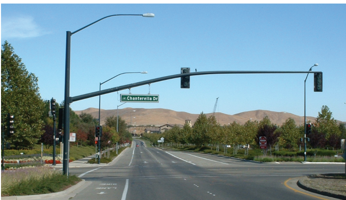
Figure 1. A typical vehicle mobility priority thoroughfare serving a single use area. Source: Kimley-Horn and Associates, Inc.
