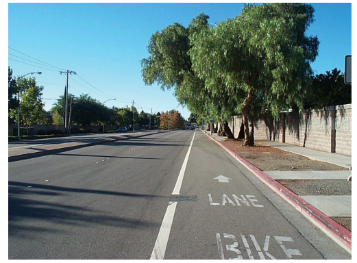
Figure 4. A wide bike lane on a mobility priority arterial without on-street parking.
