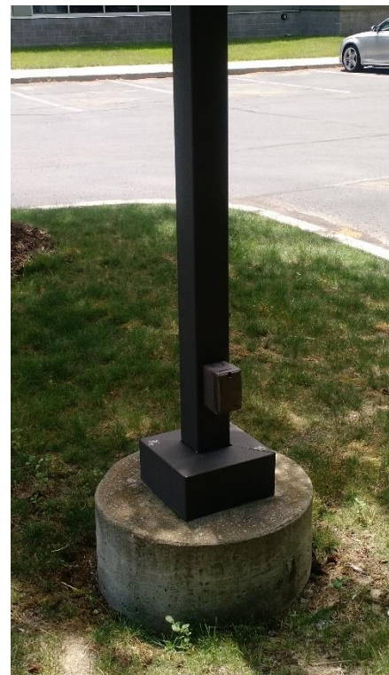
Figure 4. Outlets on several light poles at the Cornell Business Park are offered for EV charging
