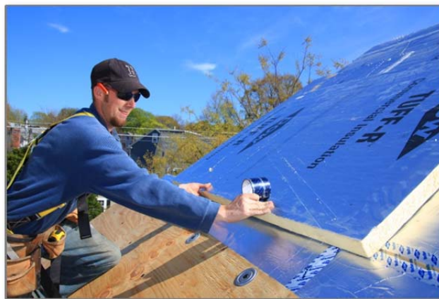
DER construction- installing roof insulation (courtesy of Dave Legg, National Grid).
