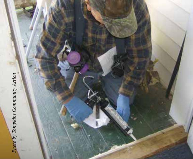
Sealing threshold of an older home, Tompkins County
