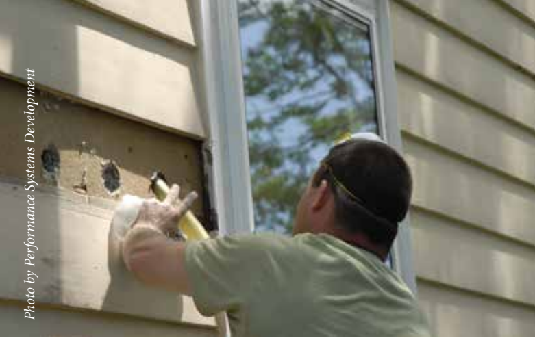
Local contractor improving energy efficiency of a house
