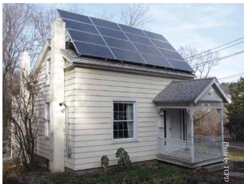
Older home with solar panels, City of Ithaca
