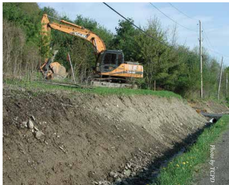
Ditch Grading in Tompkins County
