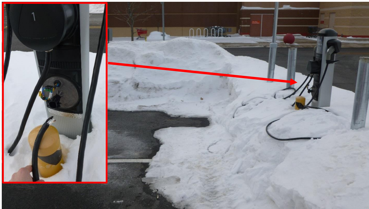
Figure 23. Charging cords not coiled up in the winter can be covered with snow and caught by a plow
