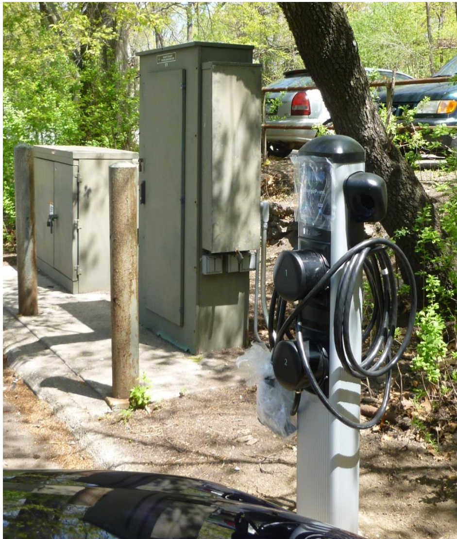
Figure 50. Charging station installation at Bronx Zoo
