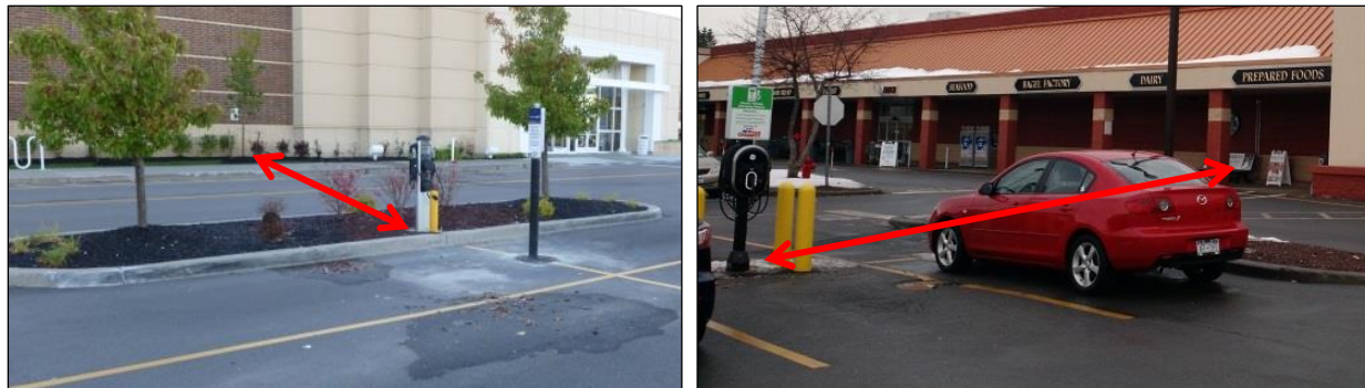
Figure 17: Charging stations at parking spaces away from a building require longer trenching through pavement and could disrupt traffic flow during construction
