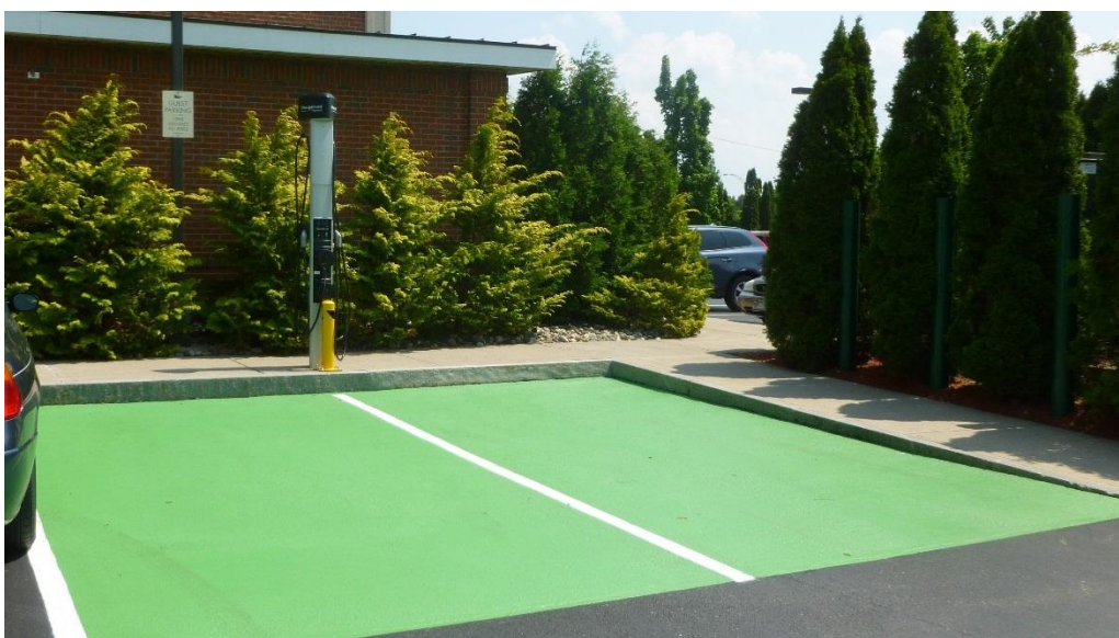
Figure 11. EV charging station space painting for easy identification
