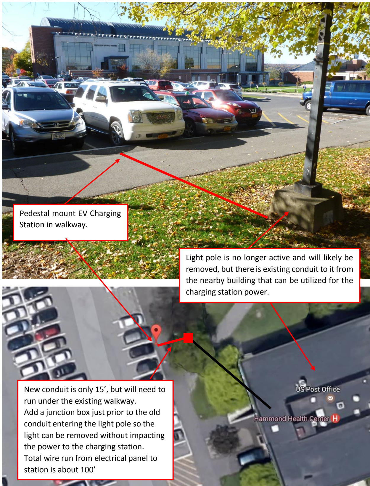
Figure 39. Electrical wiring run for the proposed placement of a new charging station at Ithaca College U-Lot
