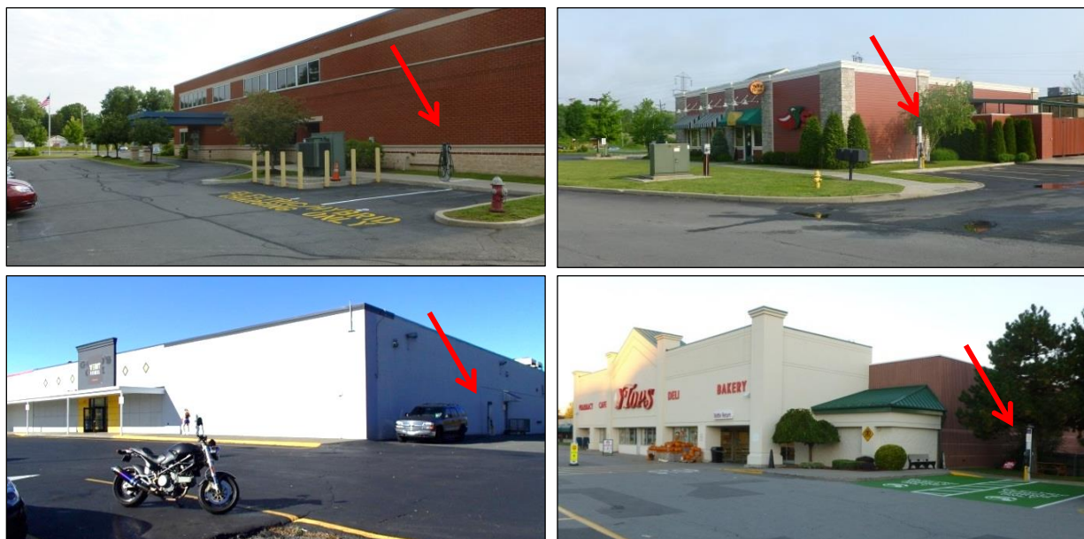
Figure 16: Charging station installations sited in convenient, but not prime parking spaces that minimize conduit runs to reduce costs
