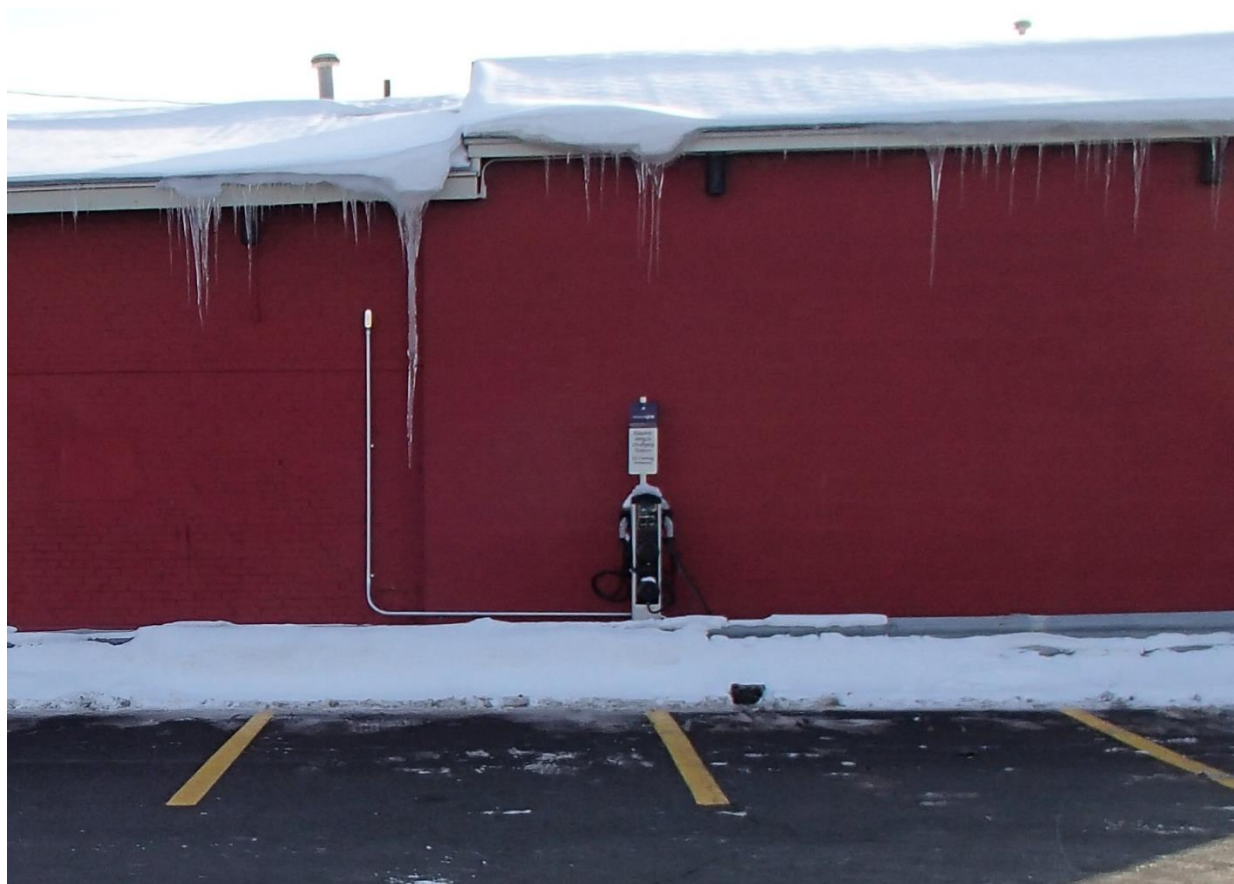
Figure 47. Charging station installation at Nichols Supermarket
