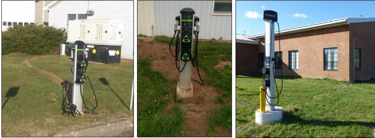
Figure 19: Examples of trenching through dirt (easiest outdoor installations)
