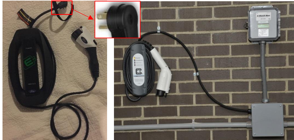
Figure 5: AC Level 1 charging cords (left) are typically sold with an EV or an AC Level 1 charging station (right) can be mounted where an EV parks
