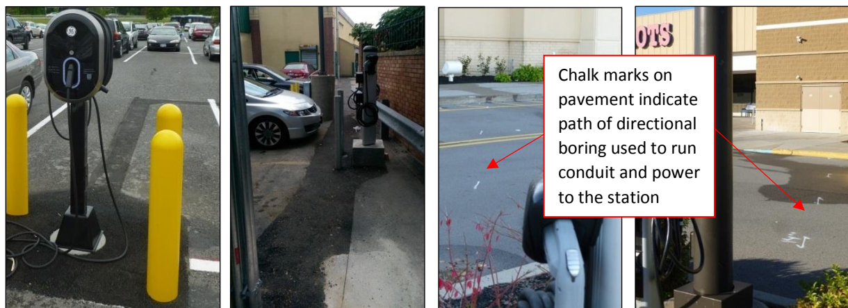
Figure 21: Parking lot pavement examples of cut/repair (left) and tunneling under (right)
