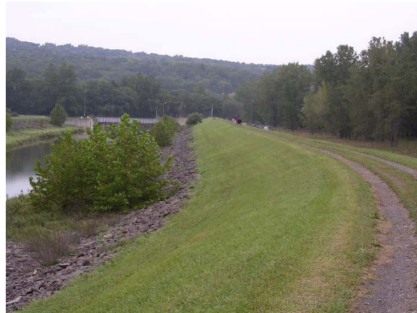
Figure 5.4.4-1. Cayuga Inlet Levee System
