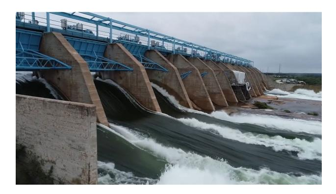
**Flood Gates**<sup>5</sup> – A flood gate is responsible for shutting out or releasing the flow of water over spillways, related to the operation of a dam. Important safety features of many types of dams, flood gates and spillways direct excess water away from the dam and its foundation to prevent erosion that could lead to catastrophic dam failure (Encyclopedia Britannica n.d.).
