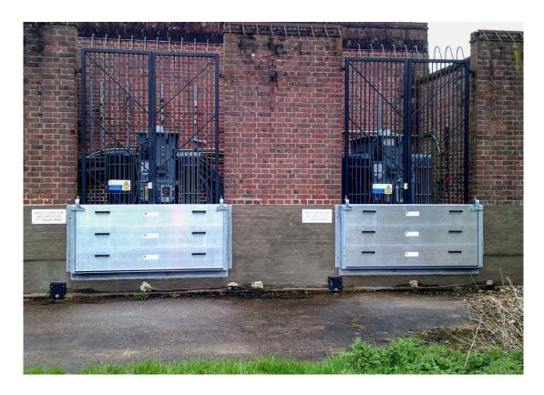
**Utility Floodproofing (Elevation and Door Dam)**<sup>2</sup> – Elevating a utility involves elevating vulnerable components of the systems by placing them on a higher platform away from flood waters. For new construction and *Substantially Improved* buildings, the most practical method to protect service equipment from flooding is to elevate above the required flood protection level, or provide dry floodproofing that protects equipment to the required flood protection level (<u>FEMA 2007</u>).
